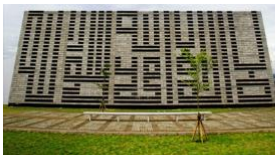
Figure 7. Facade of Al-Irsyad Mosque.
