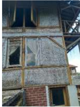
Figure 7 Openings in buildings Source: Personal documentation
