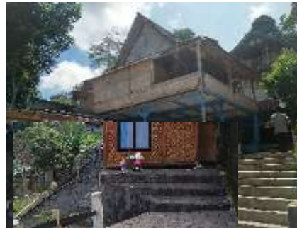
Figure 8 retaining wall of gabions in a building Source: Documentation
