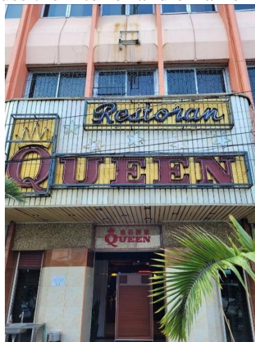
Figure 1: Front view of the restaurant
