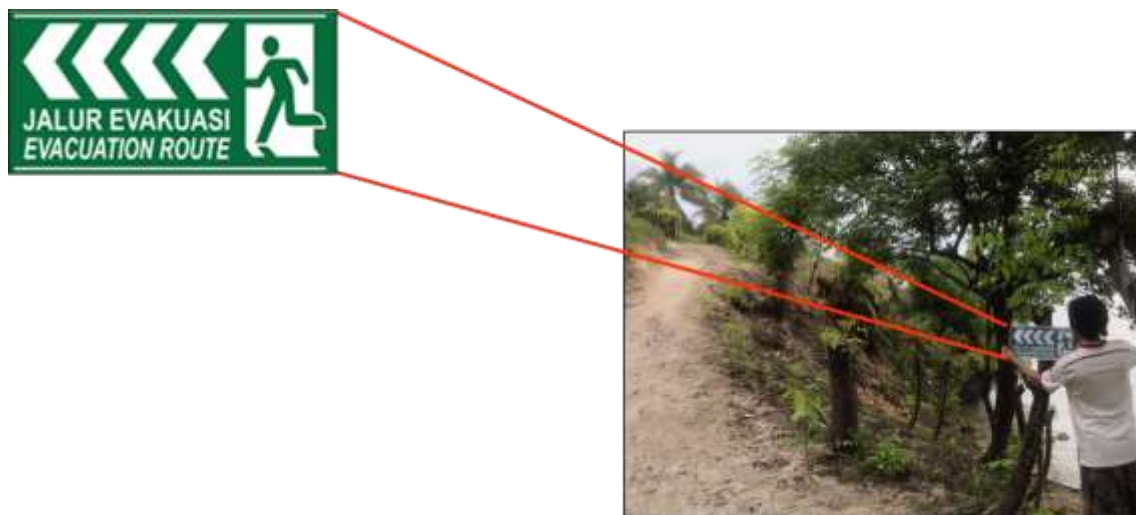
Figure 9. Installation of evacuation route boards
